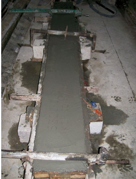
Fig. 3.6 RC T-beams after casting
