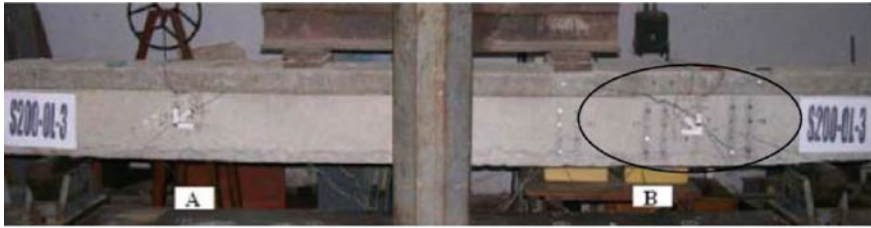
(a) Cracking Pattern of Full Beam Specimen
