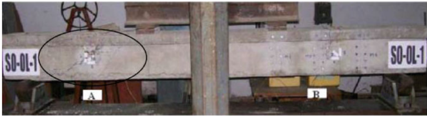
(a) Cracking Pattern of Full Beam Specimen
